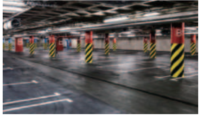
Commercial complex water drainage
