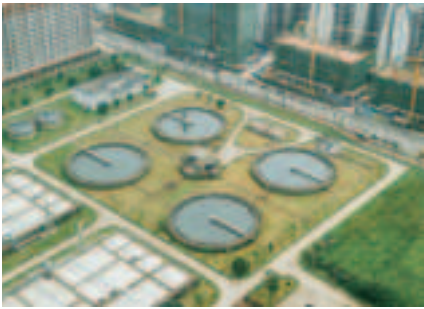
Industrial wastewater treatment
